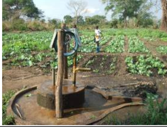
The secured water source, a lined out well with hand rope pump
