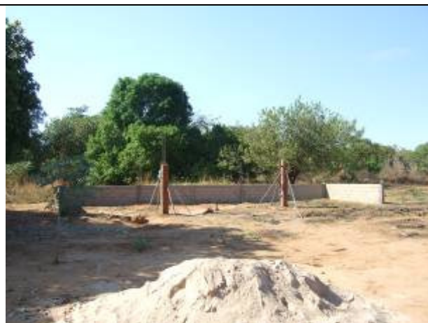
The storage shed being build, just opposite the workshop building.
