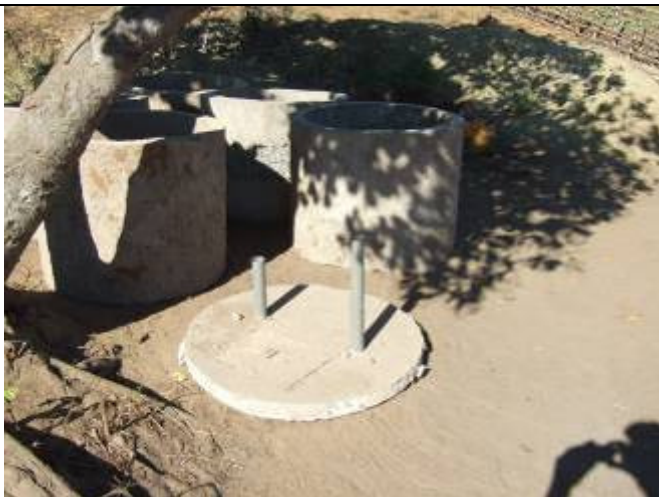
The manilha's and well cover ready to be placed
