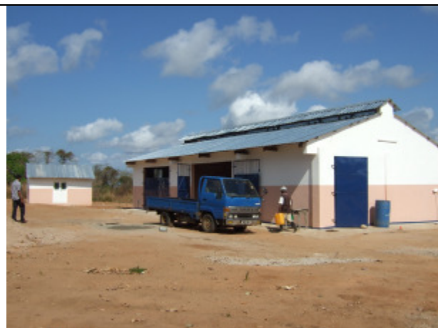
The practically completed building, with a separate generator house
