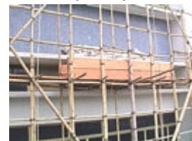
Fig. 1.3 Typical configuration of a double layered bamboo scaffold
