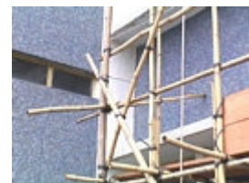
Fig. 1.5 Detail of a putlog attaching the post of the outer layer in a DLBS
