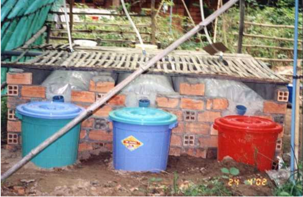
Photo 1: The construction details of each unit of three biodigesters
