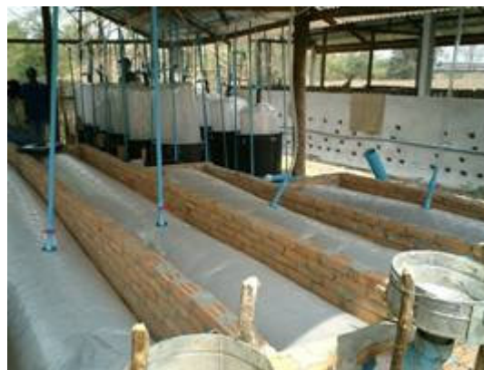
Photo 1: The construction details of each unit of four biodigesters
