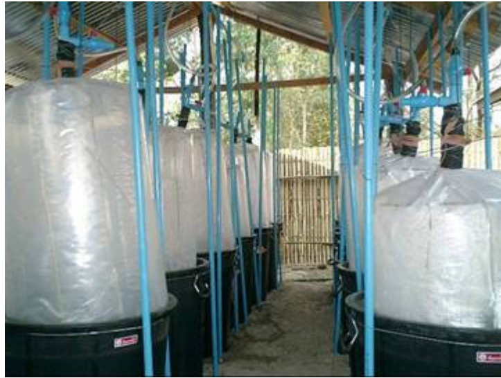
Photo 2: The inverted containers for collecting the biogas by water displacement
