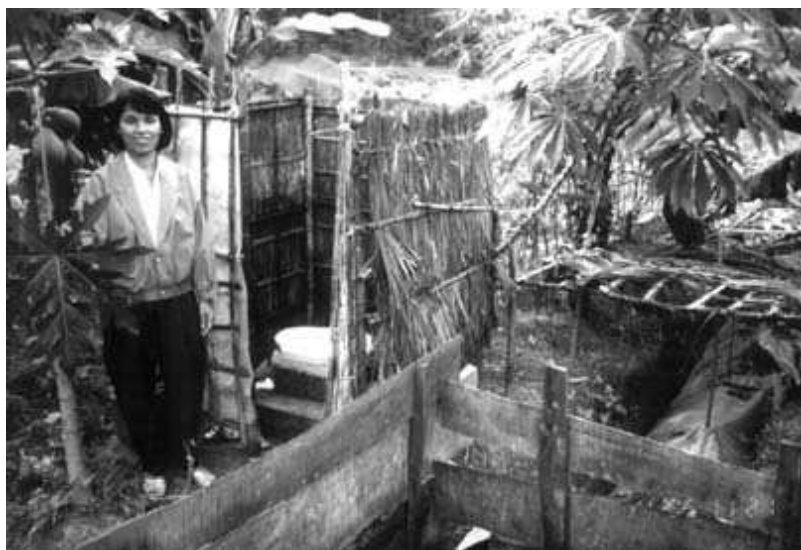
PHOTO/FOTO 9 A latrine linked to the biodigester Latrines reliées au biodigester Letrina conectada al biodigestor Photo/Foto: Lylian Rodríguez
