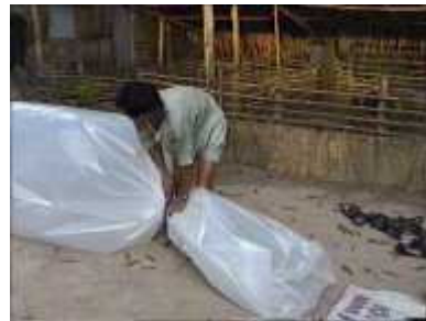
Photo 30. Tying the tube but leaving enough plastic to insert the outlet pipe
