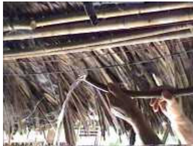
Photo 78. Accumulation of water. Open the joins and take out the water as it can be accumulated (# 6-1)
