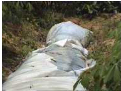
Photo 81. The outer plastic layer damaged (after 3 years..!). The inner one is still gas-tight.
