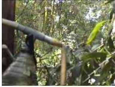
Photo 76. Hose pipe bent down (#4) Cut the damaged hose and join it again
