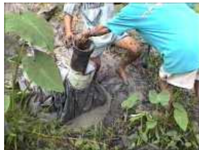
Photo 85. Pulling the plastic to one side of the trench
