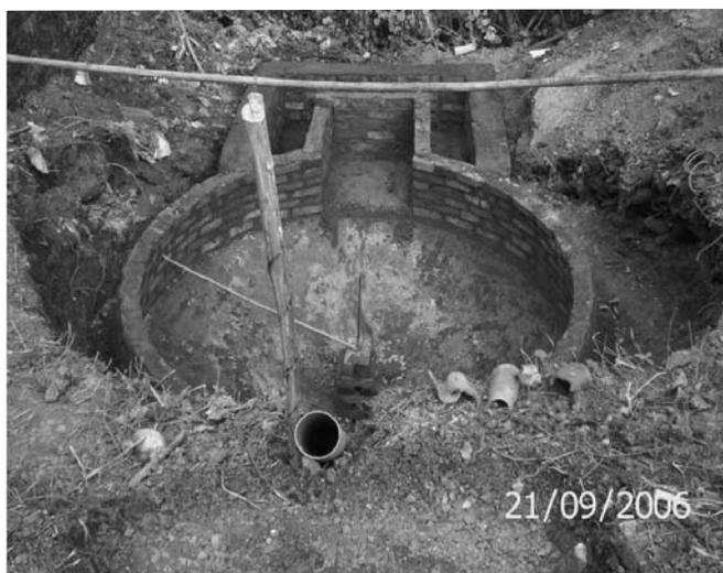
Figure 1. Digester wall construction (Photo: CV Krishna)
