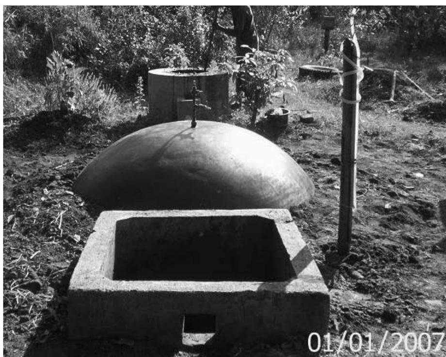
Figure 3. Biogas plant during construction (Photo: CV Krishna)
