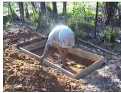
Photo 7. Placing a wooden frame (farmers can use whatever they have available, even the same mixture used for the duckweed ponds)
