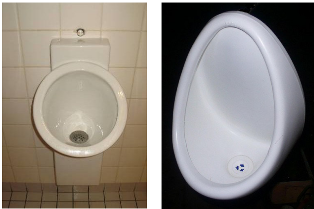
Figure 1. Waterless urinals for men (left: Centaurus model of Keramag company; right: Plastic urinal from Addicom, South Africa, with Eco-Smell-Stop device (see Table 2).
