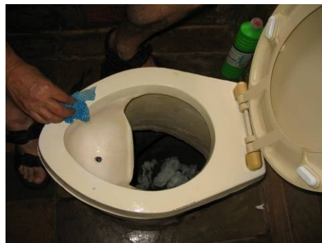
Figure 4. UDD toilet (pedestal type) in Johannesburg, South Africa at the house of Richard Holden (ecosan pioneer). Source: E. v. Münch, 2006.
