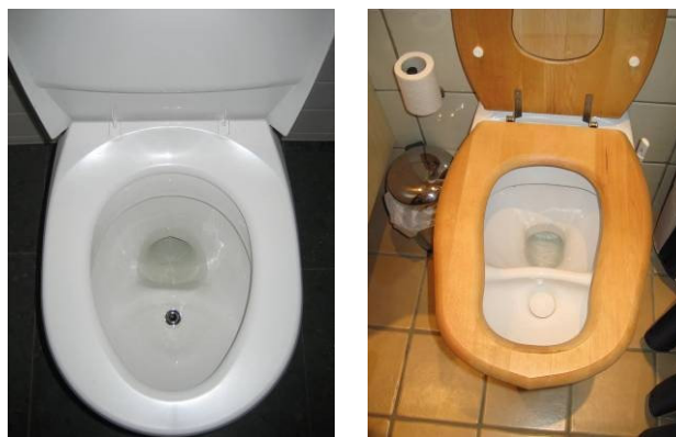
Figure 6. UD flush toilets (left: Gustavsberg (Meppel, the Netherlands); right: Dubletten (Stockholm, Sweden)). Photos: E. v. Münch, 2007.
