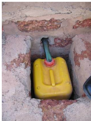
Figure 8. Low-cost solution: 20 L jerrican for urine storage at individual toilet level in Ouagadougou, Burkina Faso, Oct. 06 (photo: E. v. Münch).
