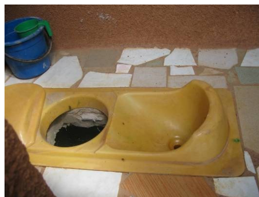
Figure 5. UDD toilet (squatting type) in Ouagadougou, Burkina Faso, installed by NGO CREPA. Source: E. v. Münch, 2006.
