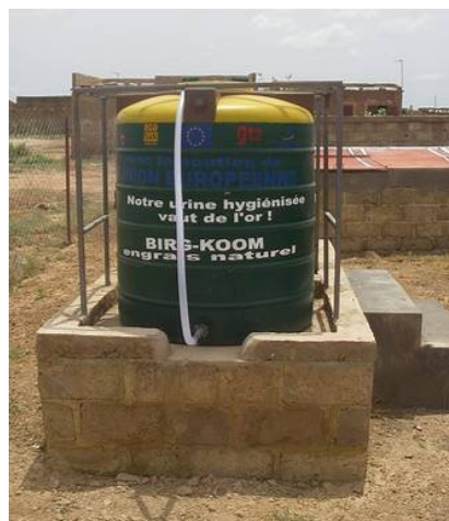
Figure 11. Above-ground plastic urine storage tank in Ouagadougou, Burkina Faso as part of EU-funded project ECOSAN_UE, Sept. 2008 (photo: S. Rüd).
