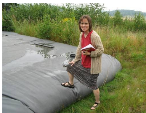
Figure 10. Urine storage tank made of a plastic bladder (3 x 150 m 3 ) at Lake Bornsjön near Stockholm (Sweden), Aug. 2007. Photo commissioned by: E. v. Münch.
