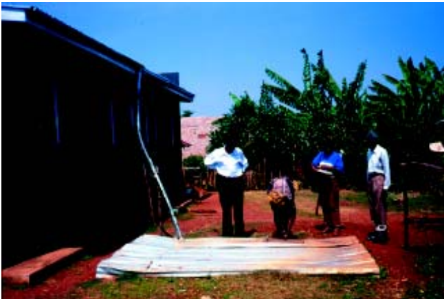
Plate 9 Roof water harvesting in Mbarara District.
