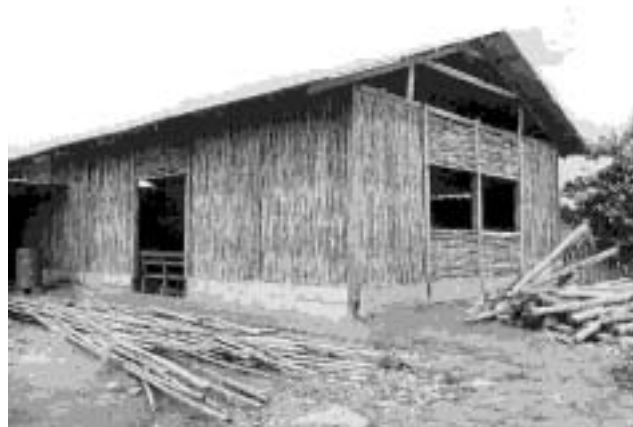
Figure 10: The Community building in Soritor during construction ©ITDG/Rumi Velacliaga
