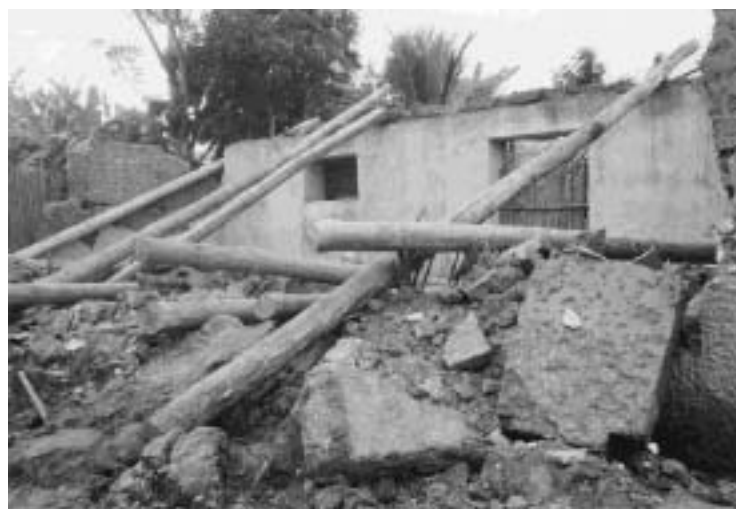
Figure 2: The impact of the earthquake on a tapial house in Soritor © ITDG/Megan Lloyed-Laney
