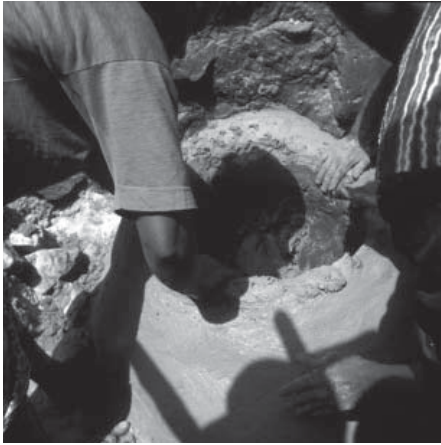
Figure 8 Final touches are given, the inside of the stove is smoothed and cleaned. (photo: Peeyush Sekhsaria)
